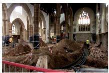
Good progress is being made. External stonework repair and restoration has been completed on the south façade, including installing four striking new grotesques high up on the parapet wall. Inside the Cathedral a limestone floor slab has been laid to create a breathable
